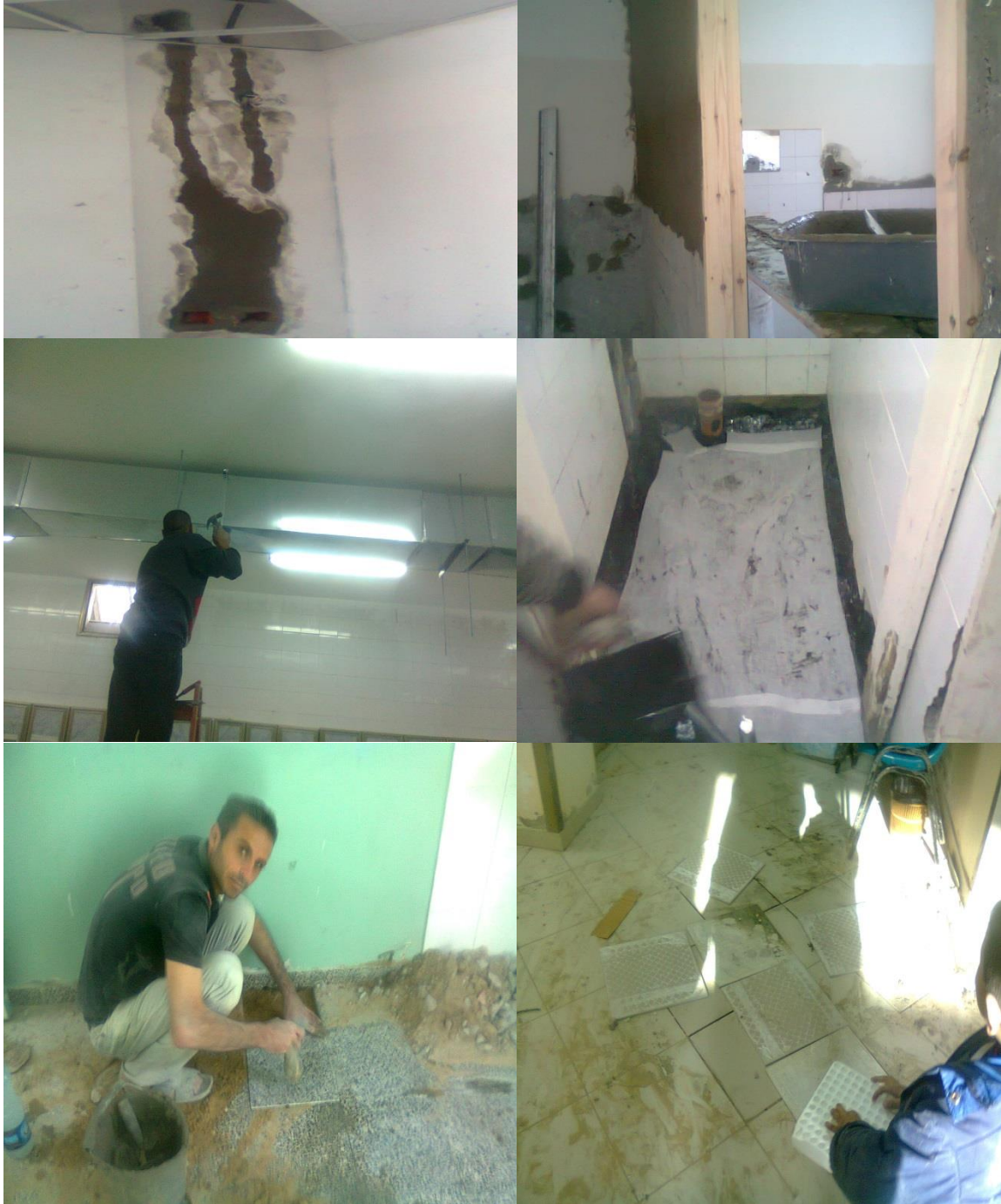
Figure 6.28: Maintain plastering and painting, HVAC, doors, windows, dooms, isolation work .
