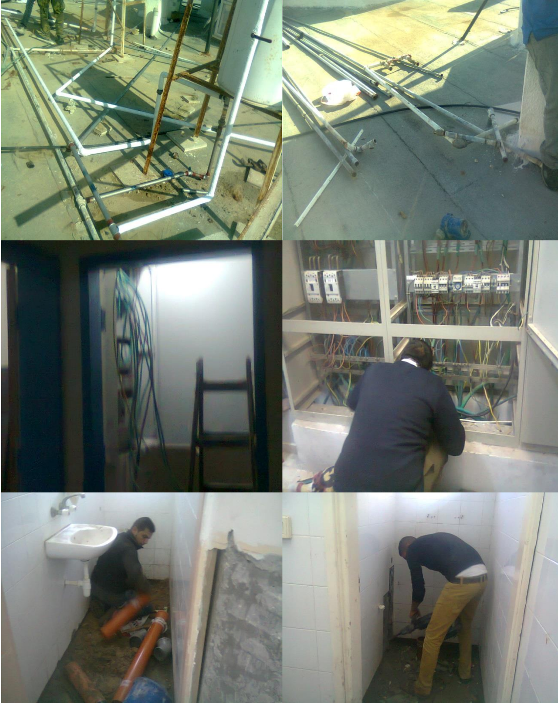
Figure 6.27: Remove electrical connections, connections before the finishing
