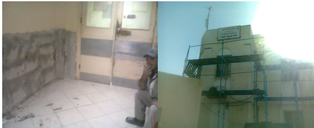
Figure 6.26: Remove plaster and painting
