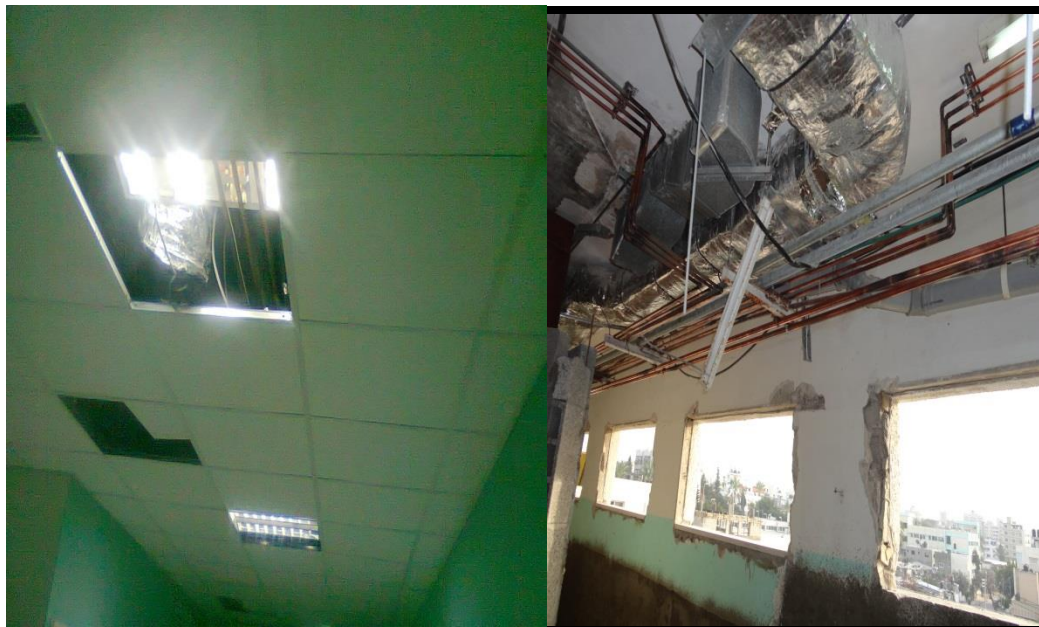
Figure 6.24: Copper pipe for medical gases pipes
