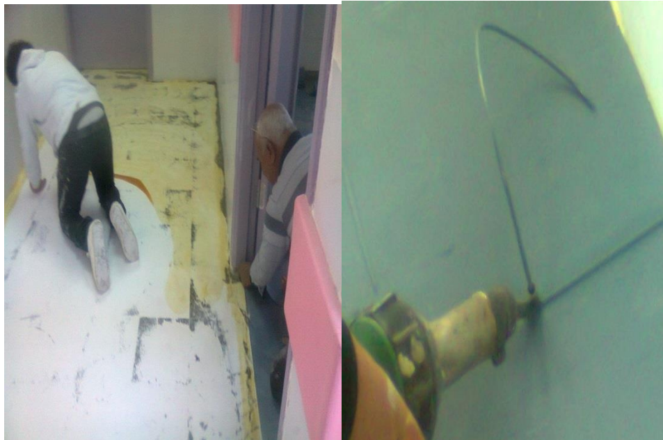
Figure 6.22: lay traflex PVC roll 2mm for corridors and rooms
