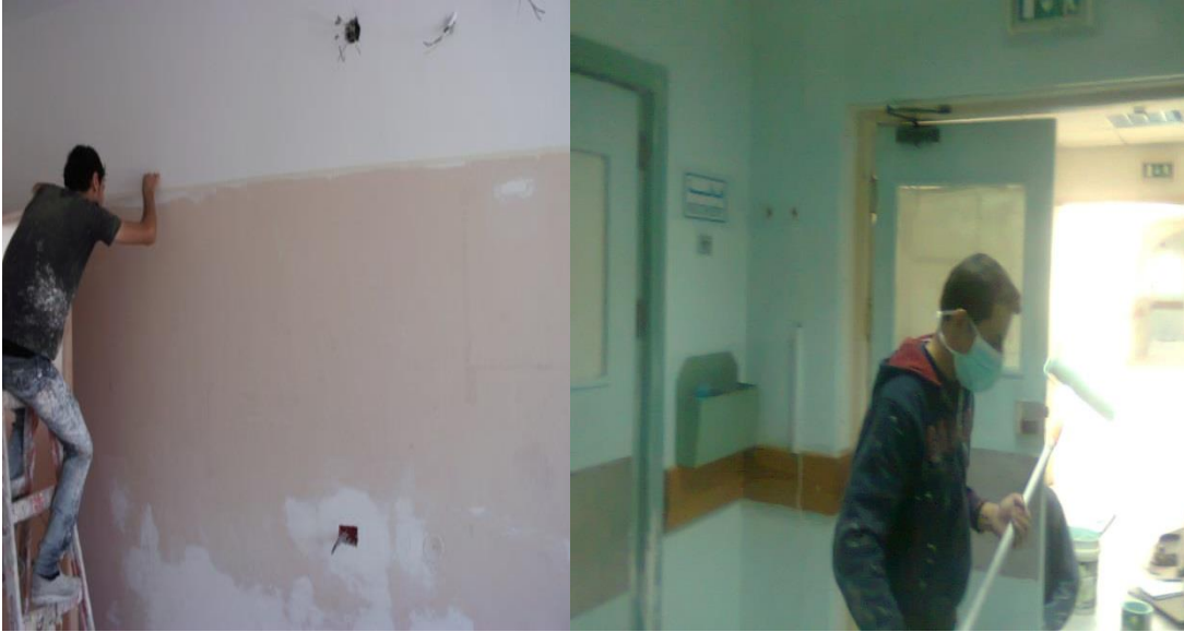
Figure 6.19: Repair any cracks and painting
