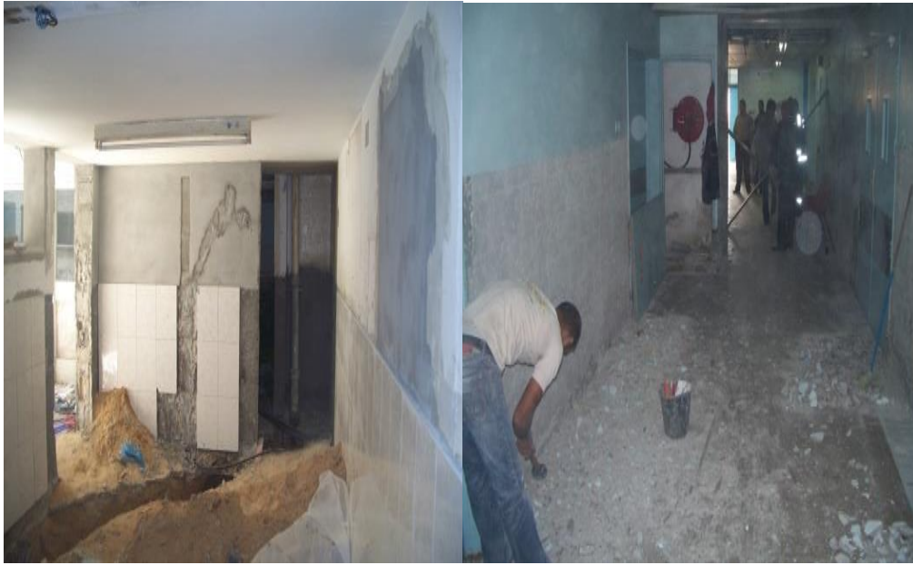
Figure 6.15: Removing existing tiles, skirting, cement and sand layers
