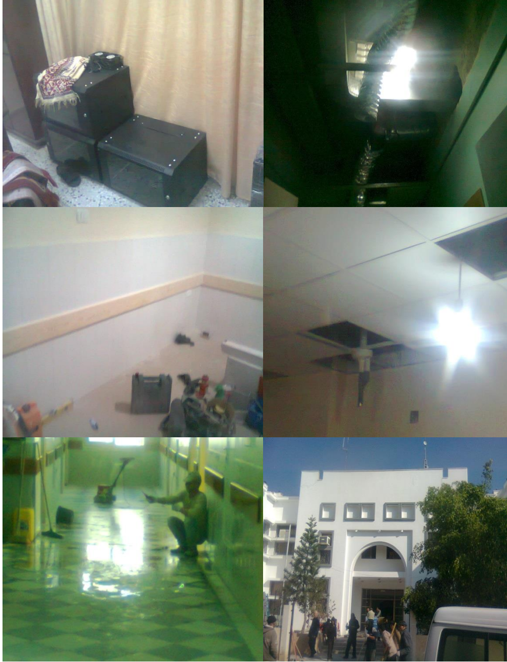
Figure 6.29: Install accessories, arms, wood protection, polish and Clean the site.
