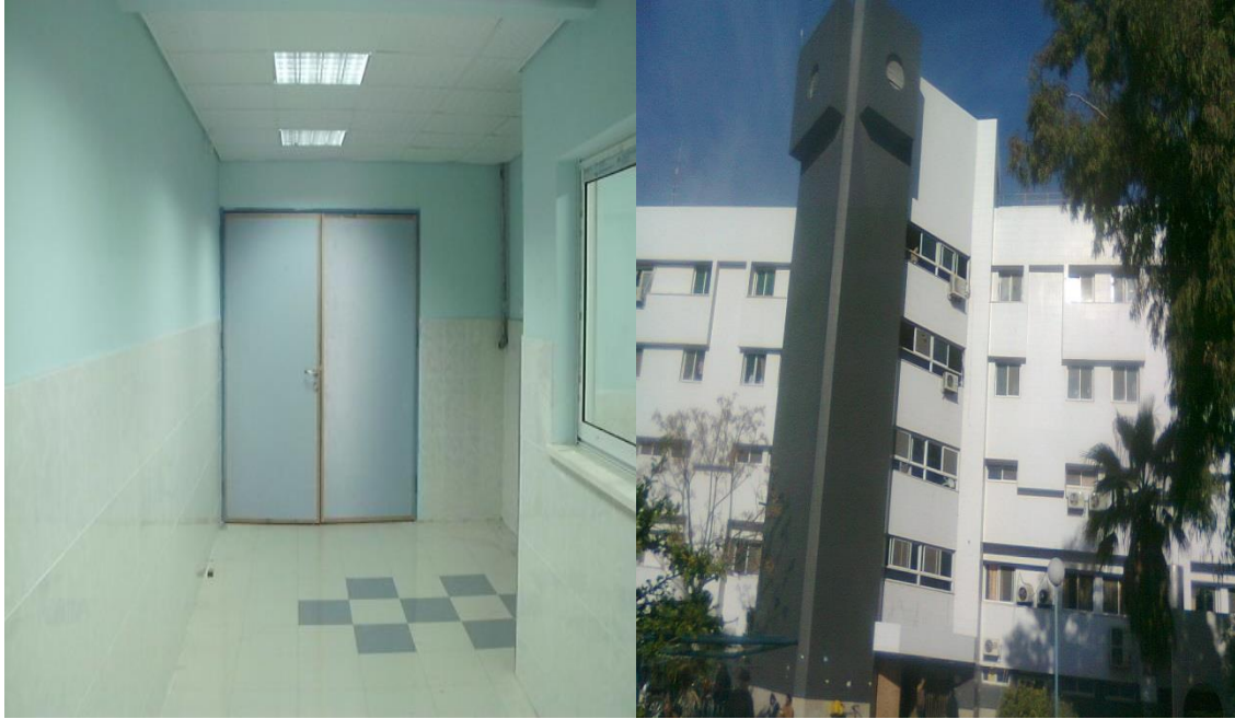
Figure 6.25: The last finish of building
