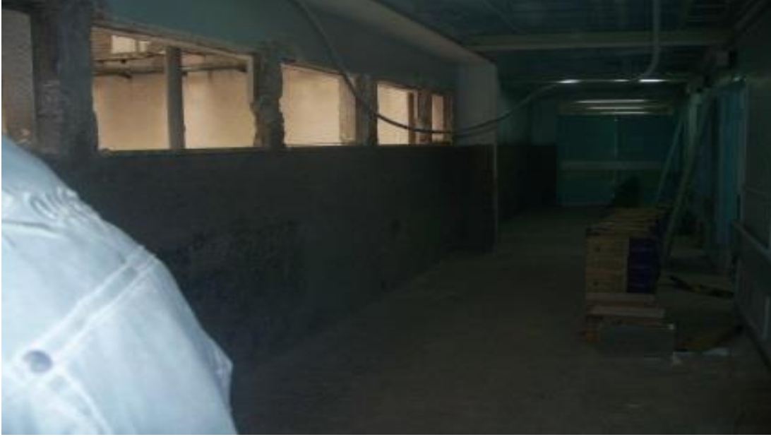
Figure 6.13: Removing existing plaster & paint from walls
