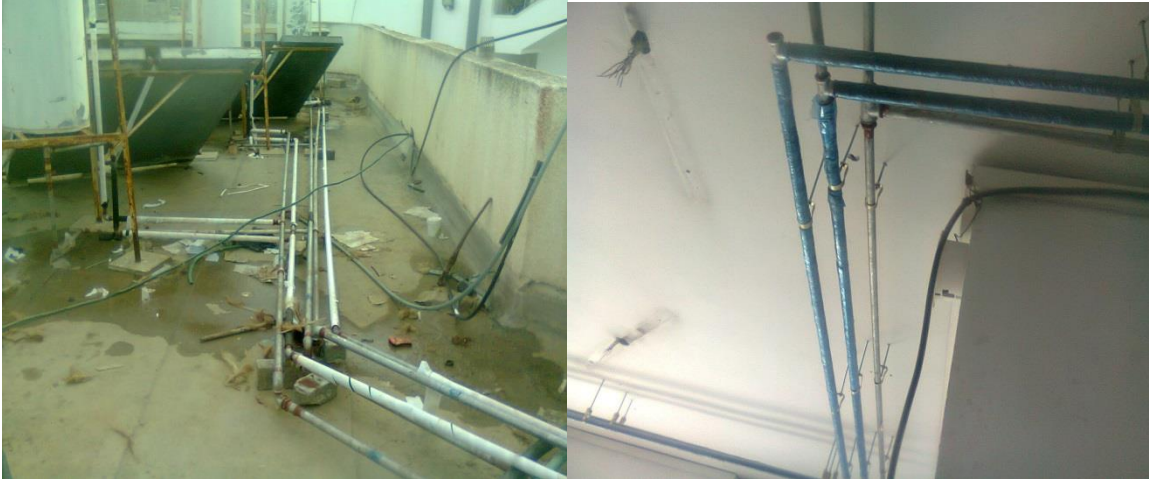
Figure 6.21: Change water network pipes with new pipes
