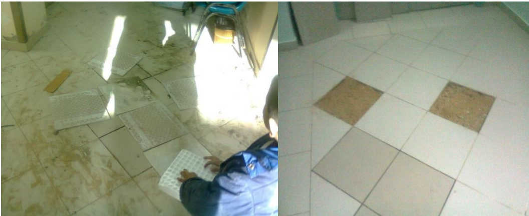
Figure 6.20: Install non slip porsolan floor tiles
