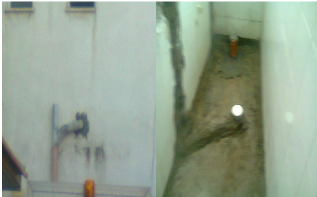
Figure 6.16: Protection concrete around sleeves and pipes
