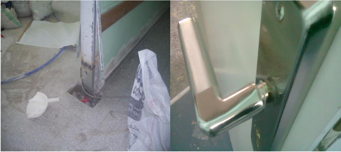
Figure 6.17: Doors shall be Italian accessories, Steel frames filled concrete
